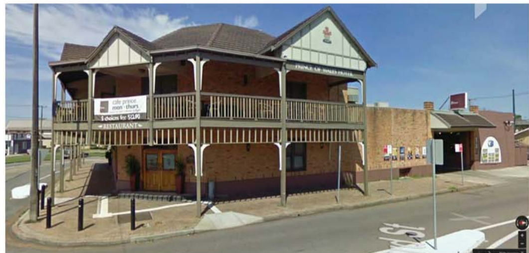
36 Lingard St. 2 Storet brick veneer Tile roof 130 metres from Subject Site
