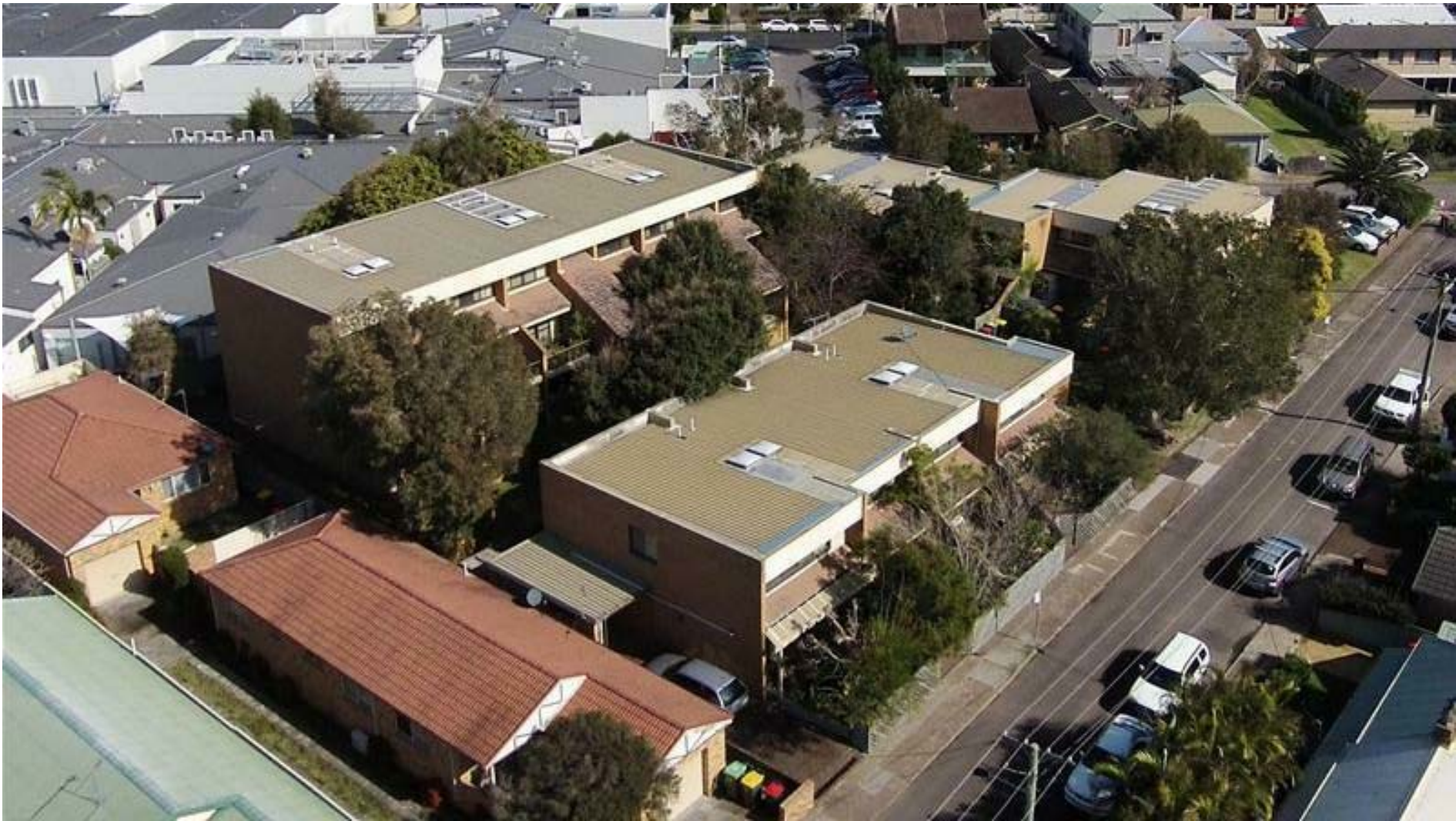
7. 1-16/27 HOPKINS STREET AERIAL VIEW
